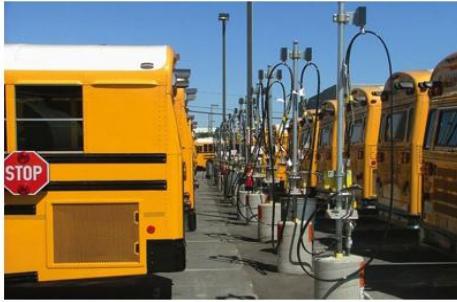
CNG Time Fill System – California
